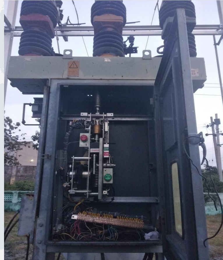
ABB-OUTDOOR BREAKER (1250A,25kA) REPLACED WITH S&S MECHANISM
