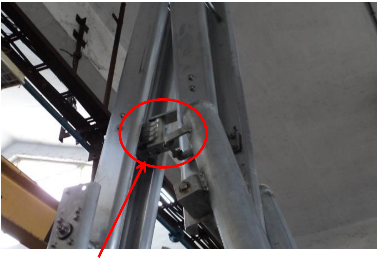
Fixed contact tube. They will be hung from the top bus bar.
